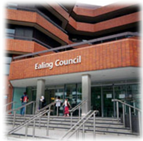
Ealing Council Offices
